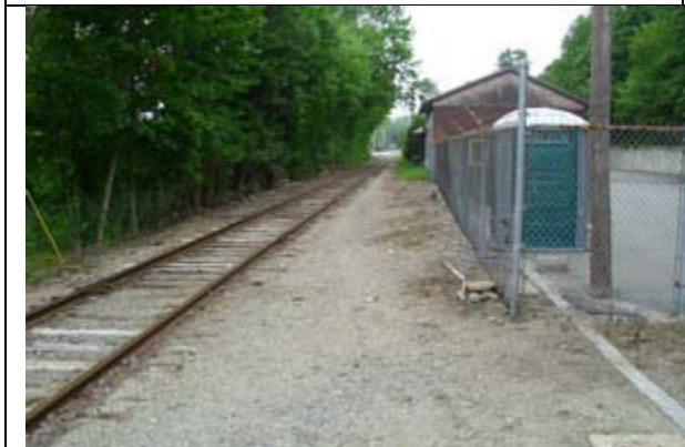
Tight squeeze between rail station and tracks
