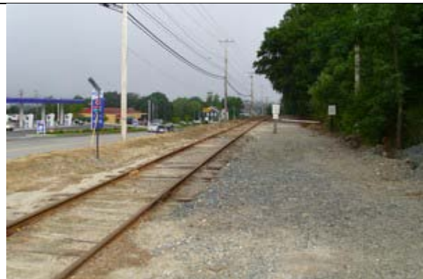
Gravel area east of tracks between rail station and Comfort Inn
