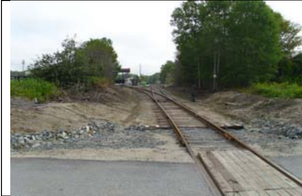
Tracks going into junction – sidings ahead
